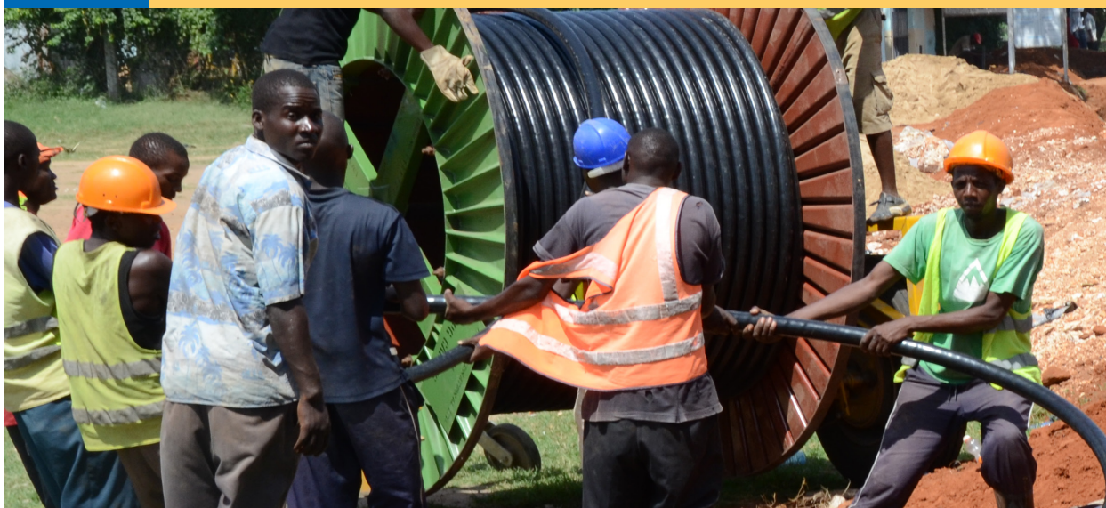
Installation of fibre-optic cables to enhance digitisation
